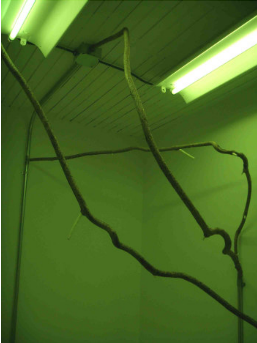
Ilene Sunshine Conduit Detail Location: Alcove Annex
